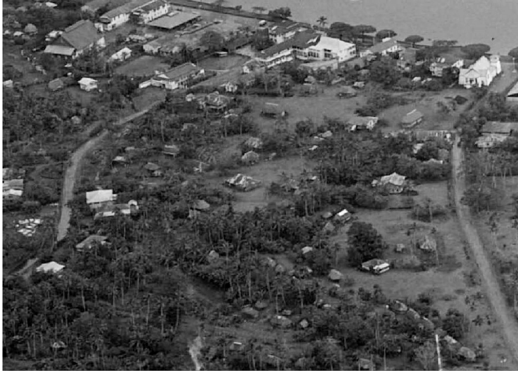
Figure 6: Close up aerial photograph of the Project field site.
